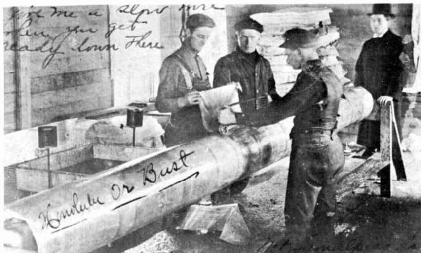
PW technicians winding a helix coil for the Mt. Tamalpais station; Mr. Krenke at far left. Cloth stacked in corner was applied over each layer of wire and coated with shellac. Process was not unlike that used for making today's surfboards with fiberglass.
